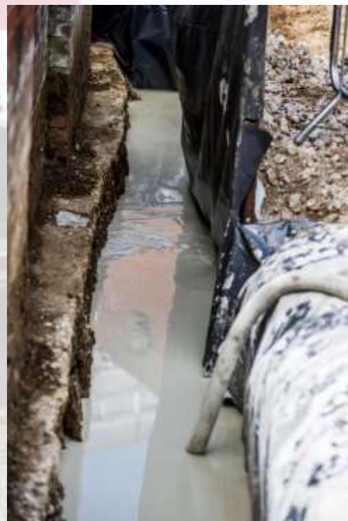
Infilling cut off wall sealing contaminated land.
