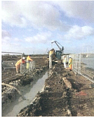
Slurry wall infill
