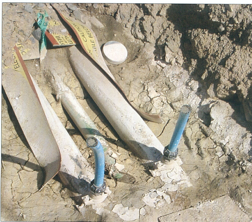
Photograph Above. Bentonite being applied
