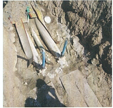
Infilling underground electric cable ducts
