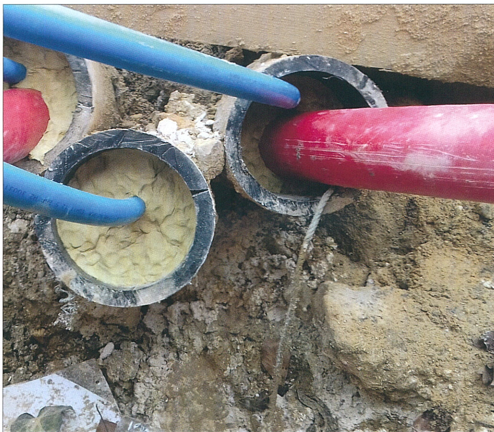
Photograph Above. Infilling of electrical cable ducts
