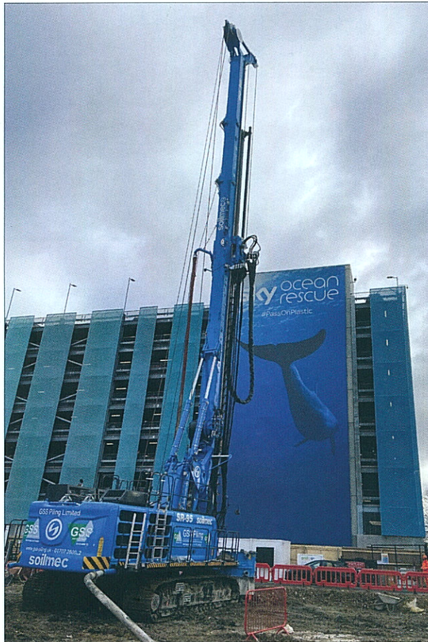
Photograph Above. Bentonite can be used on secant pile walls (soft piles) typically specified as 0.7-1.0 MPa after 28 days and geothermal piles
