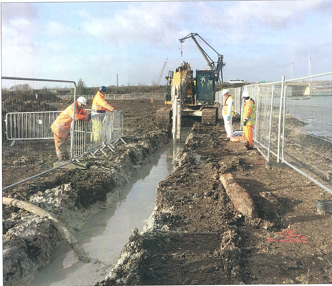
Photograph Above. Infilling of cut off wall sealing contaminated land
