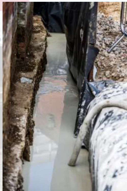
Infilling cut off wall sealing contaminated land.
